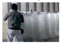
2. Double sided tape: First, apply tape to container walls. Second, peel off tape backing. Lastly, unroll SideGuard against the wall (Foil Facing In).
